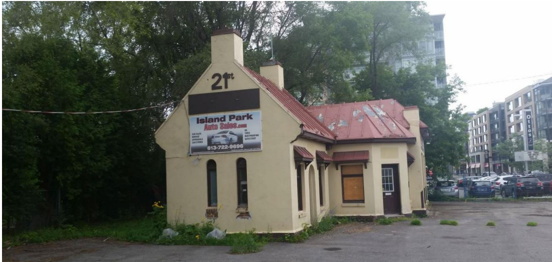
Figure 11: Contemporary view of the Service Station from the east. Source: City of Ottawa Designation File.
