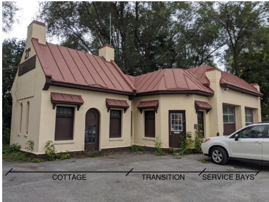
Figure 28: View of building referencing the house-form commercial section, the adjoining office area, and the two-bay service section.
