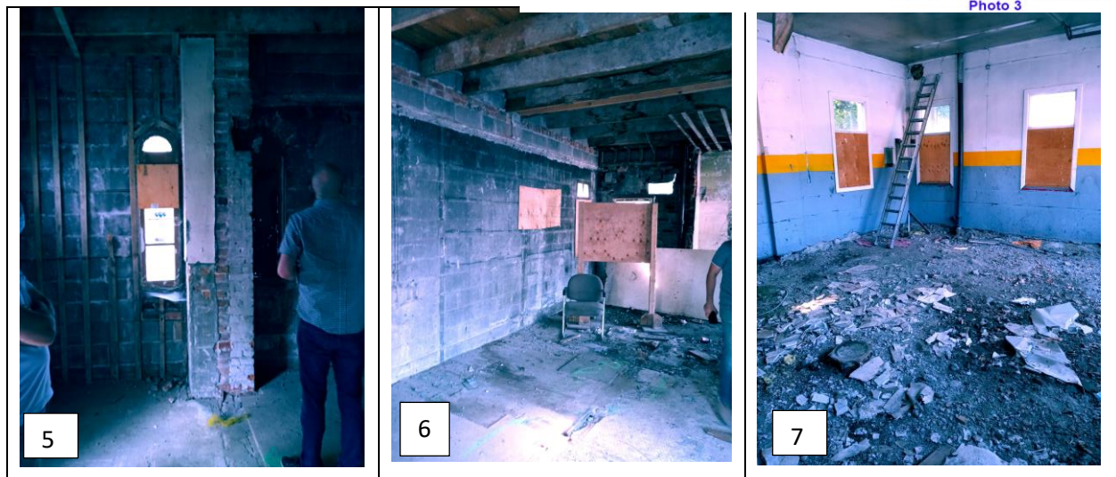
Figure 20: Interior views; 5. Looking towards the east wall with round headed windows on either side of the chimney. View 6. And 7. Interior views of transition area and the service bays. Source Commonwealth 2021
