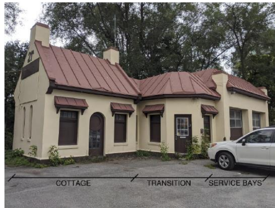
Photo 1: Overview of building [JCAL 2020]
