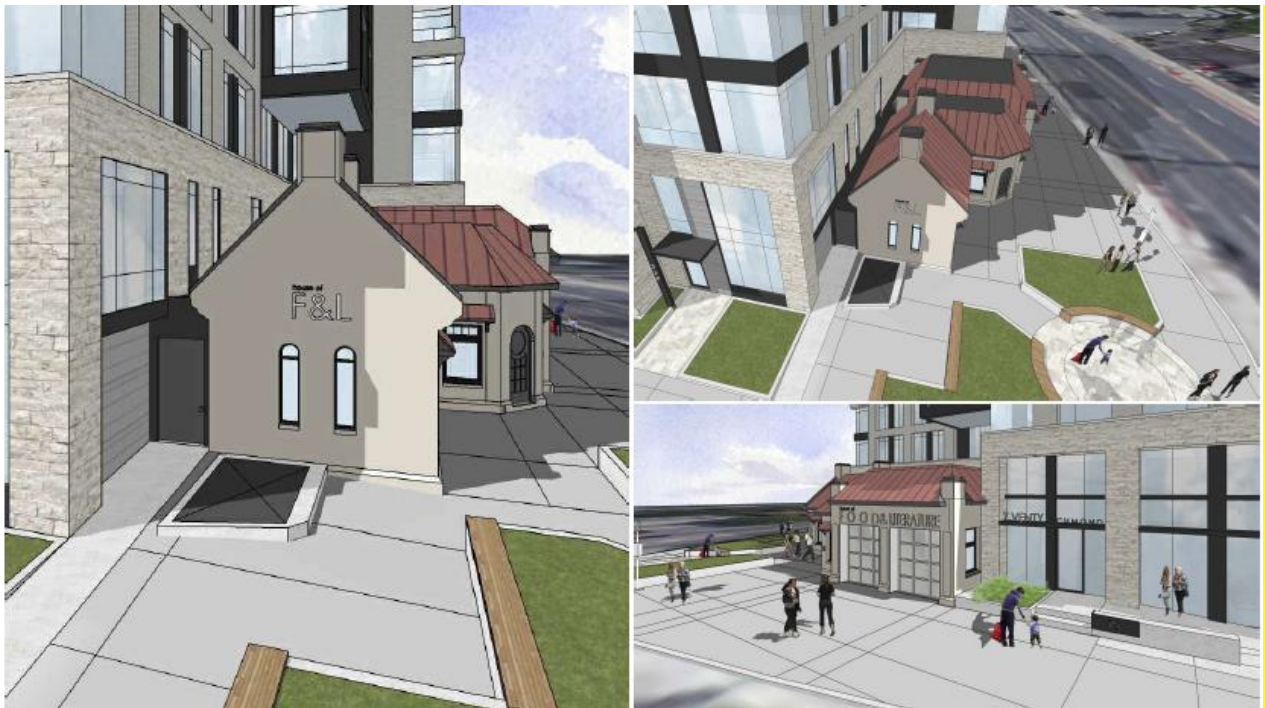
Figure 10: Views clockwise - 1. from the west illustrating the recessed link between the Station and the apartment, 2. Aerial view illustrating the massing and ability to interpret the entire building as a separate feature. 3. A view looking south east illustrating the side window. Source: Hobin architecture 2023.
