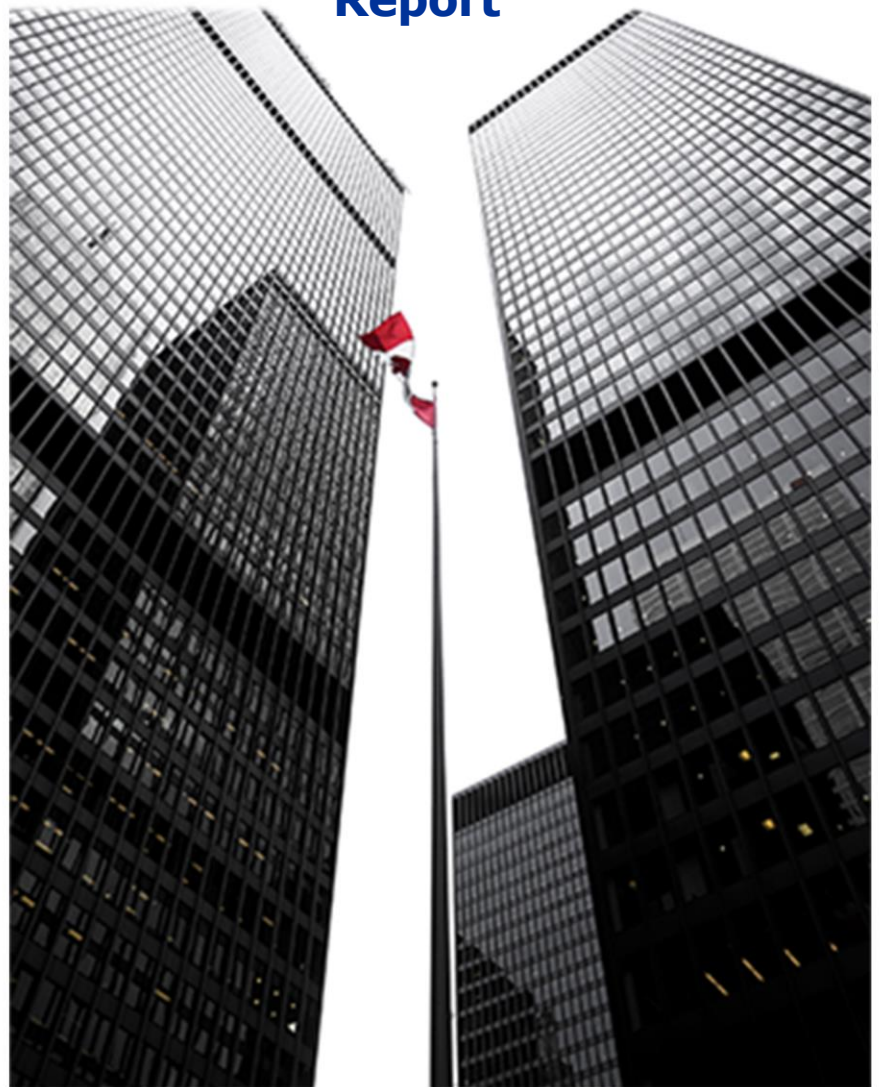
Project: 70 Richmond Road Devtrin (Island Park) Inc.
