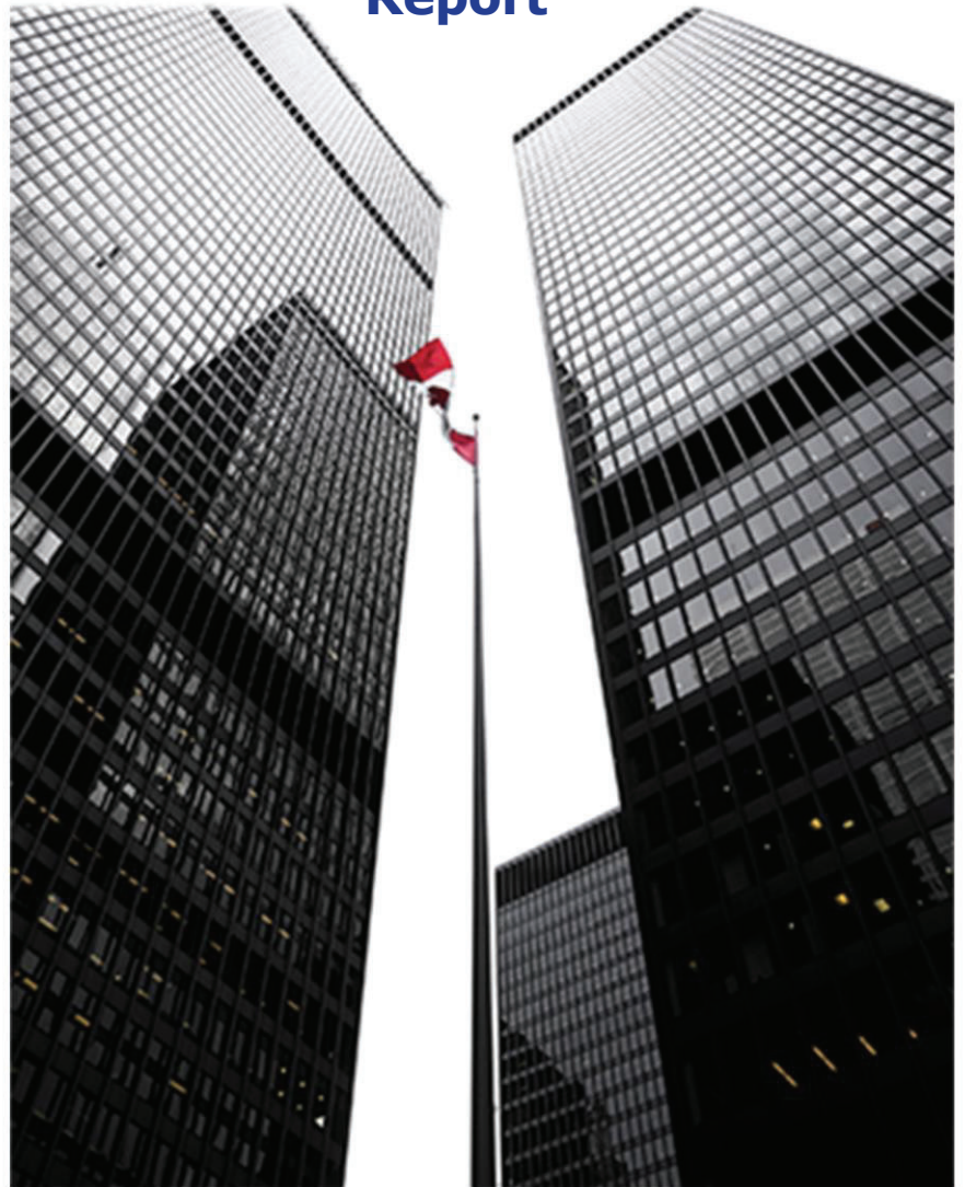
Project: 70 Richmond Road Devtrin (Island Park) Inc.
