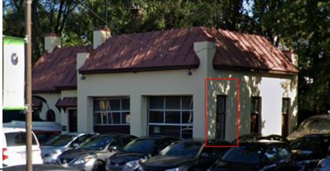
Figure 22: This view highlights in red the first of the three windows along the west side of the Service Station. The proposed midrise building has been set back and allows the side window to be interpreted from the exterior. Source: City of Ottawa.
