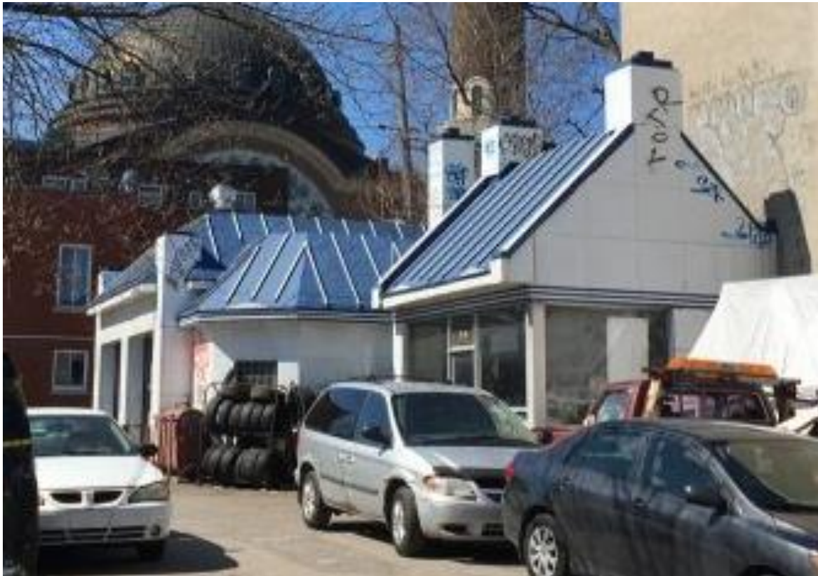
Figure 2: Former Champlain service station, 55 Saint-Viateur Street West Montreal is a mirror image of the Service Station at 70 Richmond Road. Source: [photo: Justin Bur 2017]
