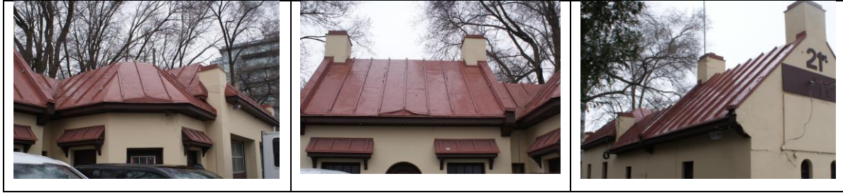
Figure 3: images of the Roof
