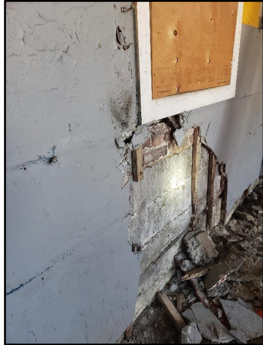
Masonry Wall Behind Plaster Lath - Service Bay
