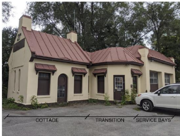
Photo 1: Overview of building [JCAL 2020]
