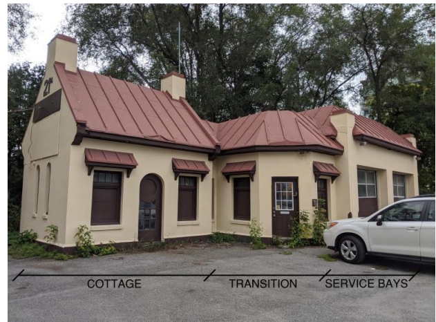
Figure 1: View of the Service Station with the 3 sections cottage, transition, and service bays.
