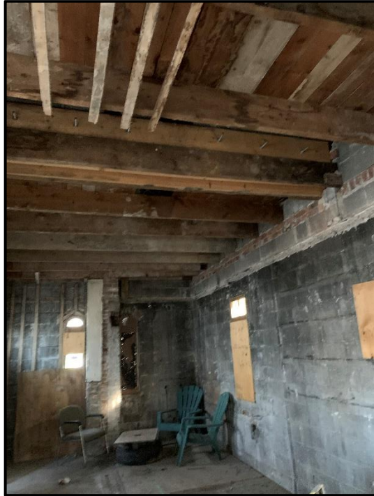
Roof framing administration area
