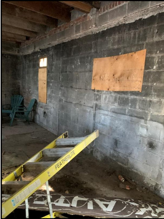
Exposed Masonry Wall Administration Area
