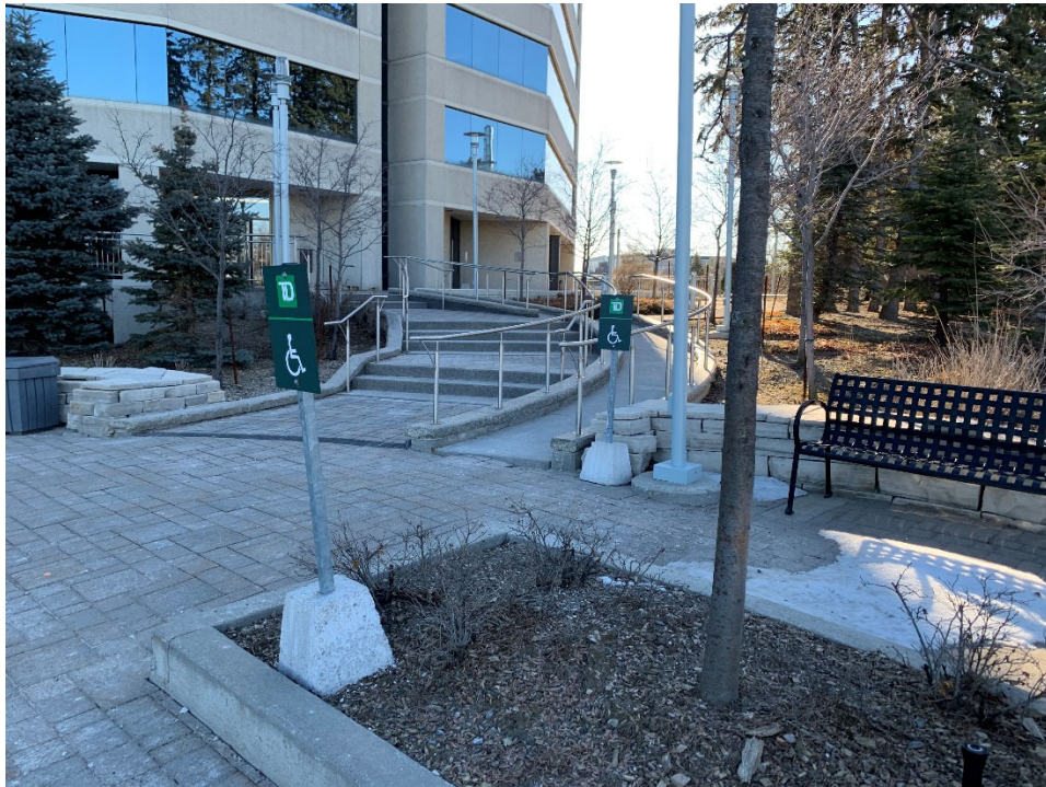
Photograph 5 – West entrance and ramp
