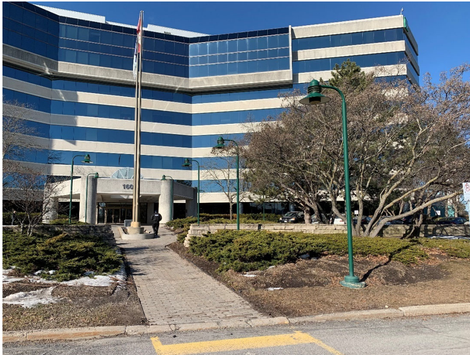
Photograph 1 – Main walkway leading to East Entrance
