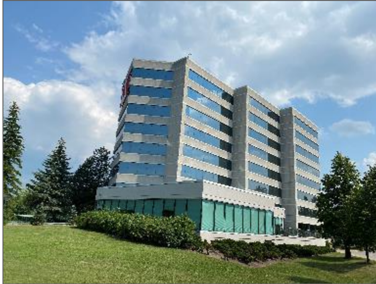
Photo 1 – Site Building (north elevation).
