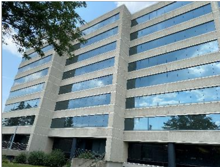
Photo 4 – Site Building (west elevation).
