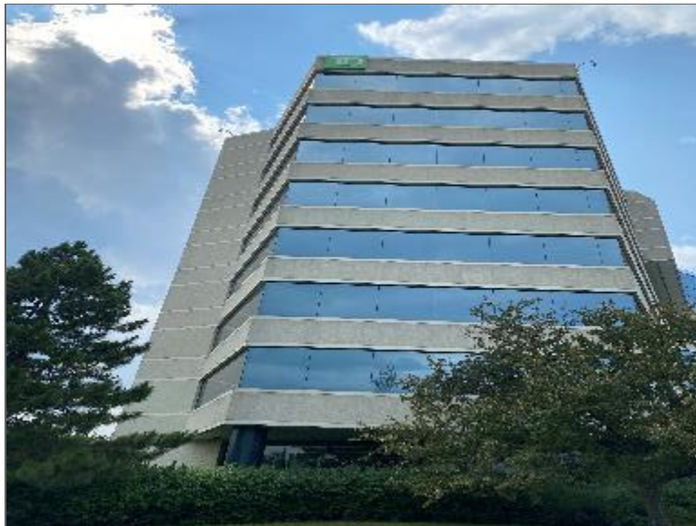
Photo 2 – Site Building (south elevation).
