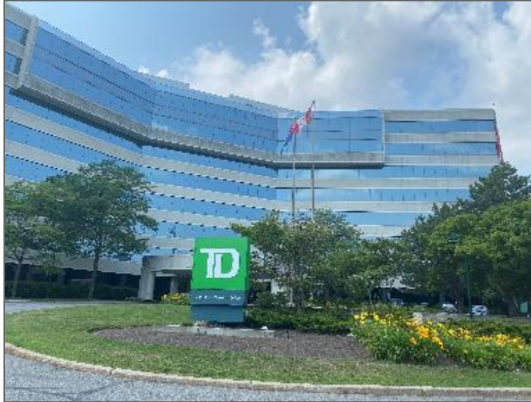
Photo 3 – Site Building (east elevation).
