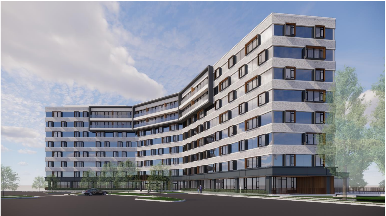
Figure 8: View looking south towards the Phase I conversion
