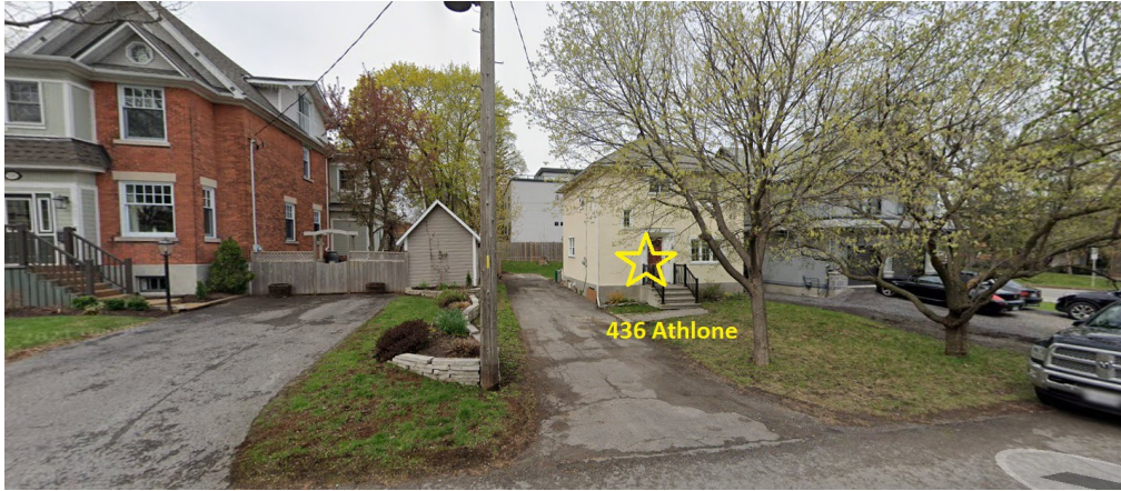
Image 5.1 – view from the street looking at the existing home at 436 Athlone
