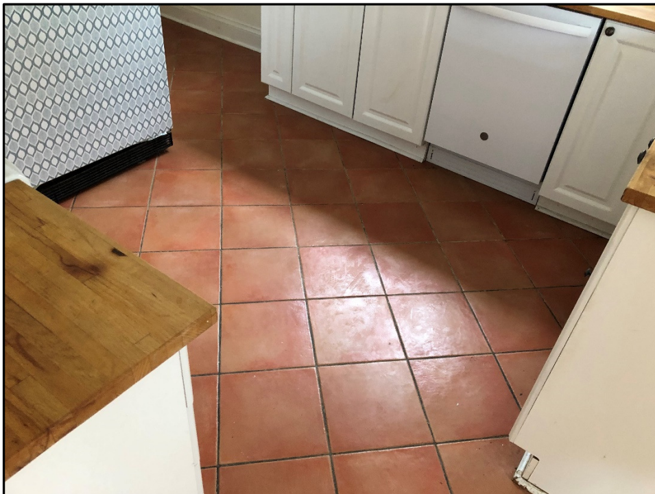
Photograph 2: Ceramic tile flooring in the first-floor kitchen.
