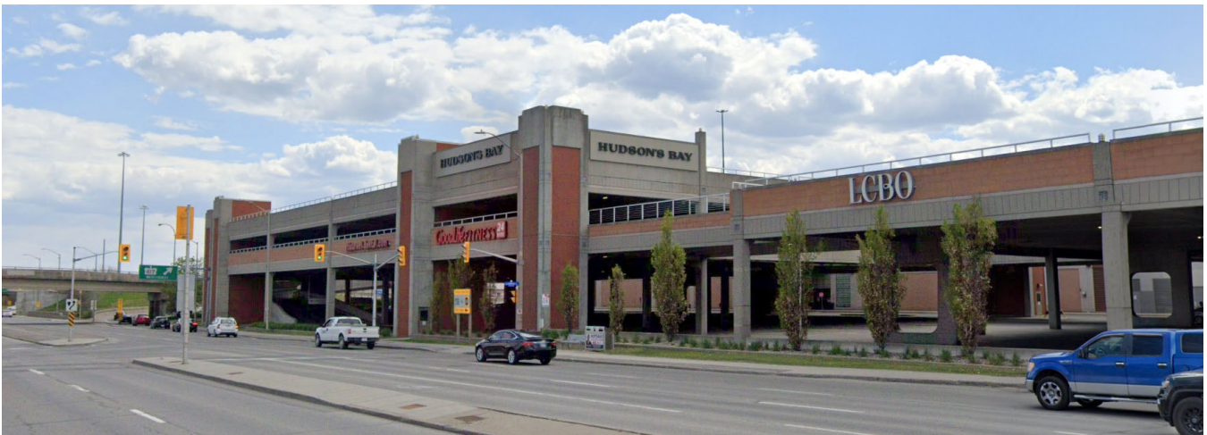
Figure 5: View of St. Laurent Shopping Centre Parking Garage from St. Laurent Boulevard
