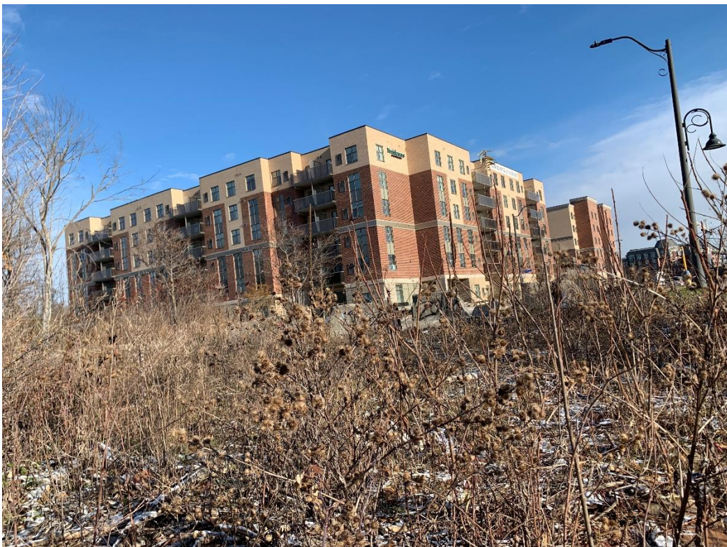
Photo 8: Commercial property located northeast of the Site.
