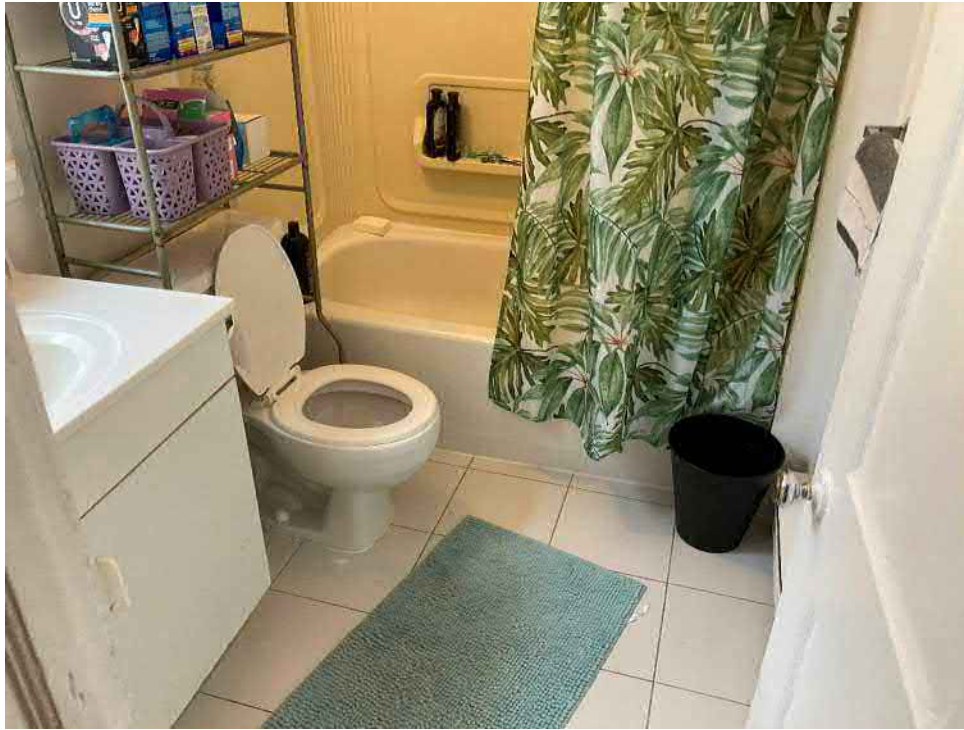
Photo 13: View of the bathroom on the second floor of the building.
