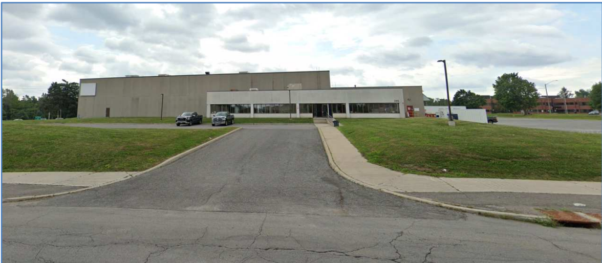
Existing Site Conditions: Facing South
