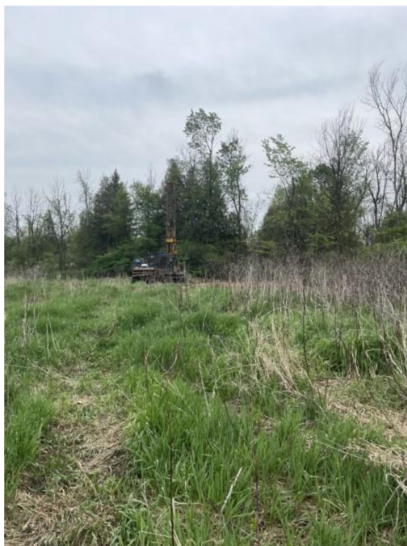
Photo B: Geotech
