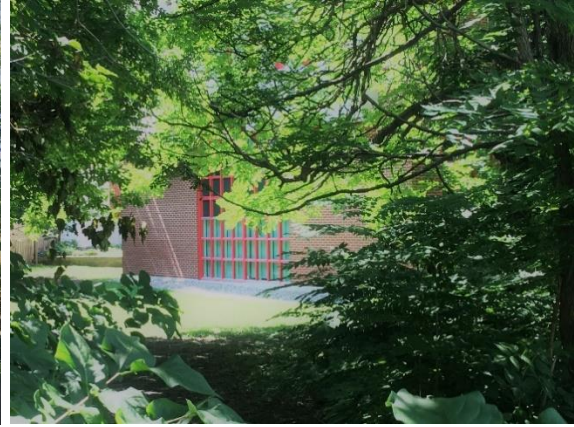
South facade Photo: City of Ottawa, August 2020
