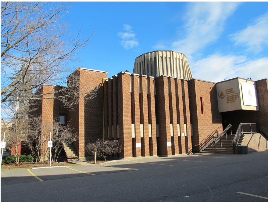
Rear elevation (1966 building)
