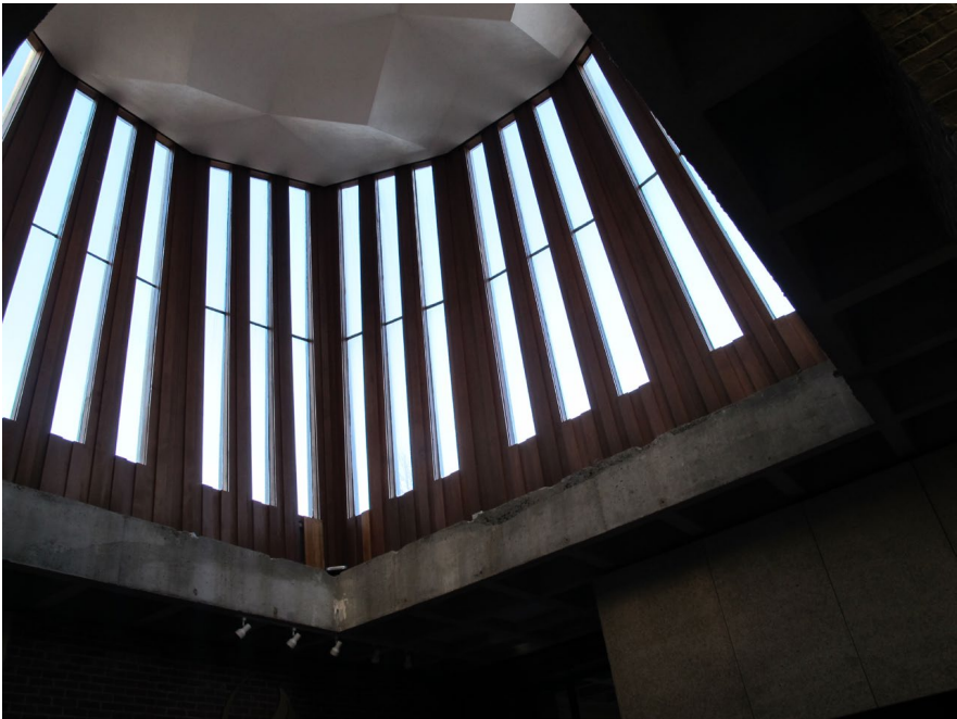
Underside of lantern
