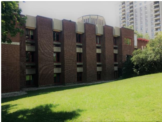
East façade, looking north west Photo: City of Ottawa, August 2020
