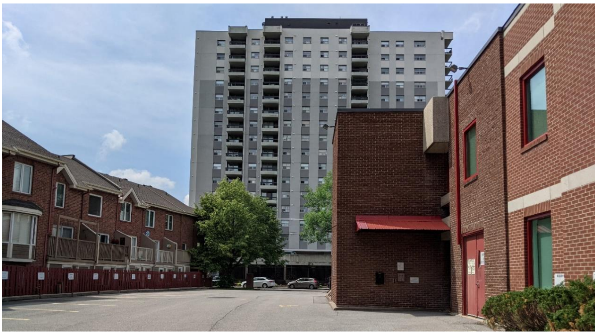
Figure 17: From existing parking lot of adjacent 17-storey Tower (40 Driveway).
