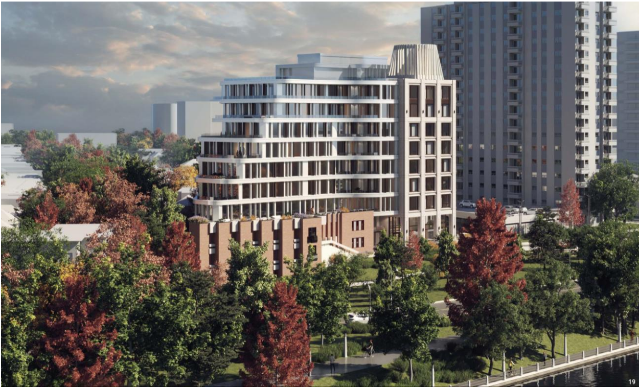
Figure 1: Redevelopment proposed at 50 The Driveway. Source: Hobin Architecture Incorporated
