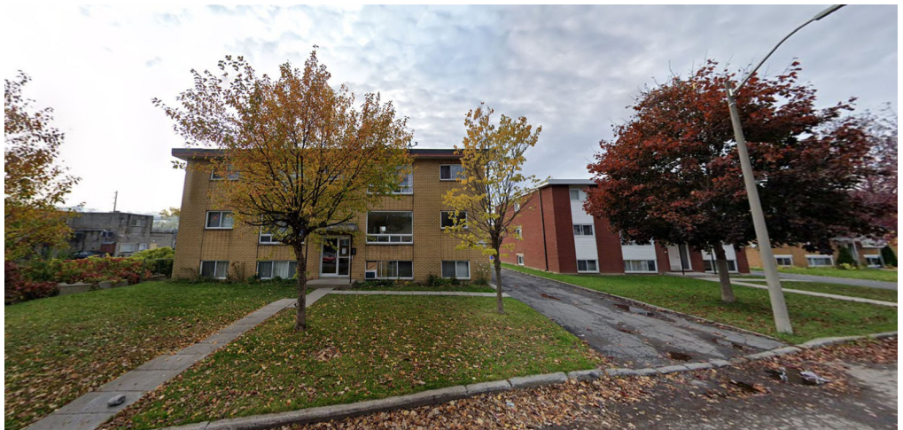
Image 03. Adjacent property to North of site.
