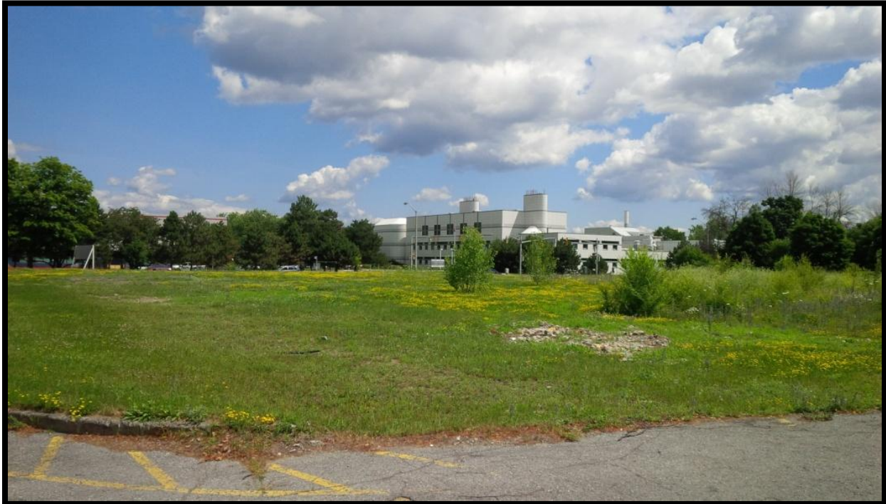
Photograph 1: View of the east side of 770 Brookfield Road. This area was the former location of a multi-storey office building, now a grassy field with exposed rubble. Looking northeast. Office buildings can be seen in the distance.
