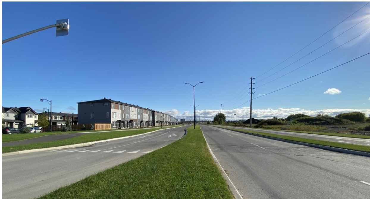
Figure 5: The existing road conditions and public realm of Campeau Drive
