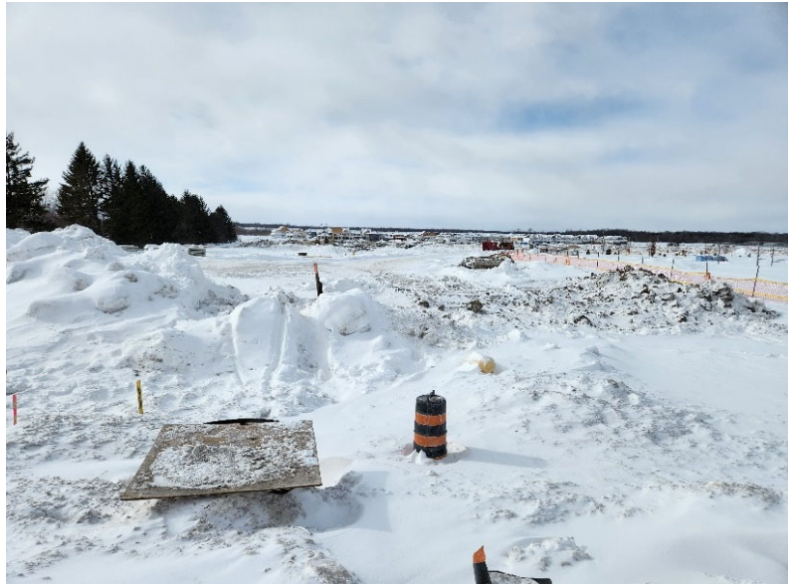
Photo 1 - Looking west across the Site, from Bank Street
