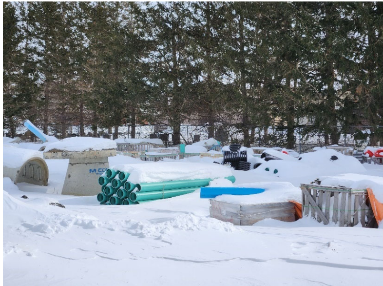
Photo 4 - Construction materials stoed on-site
