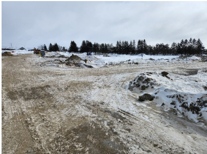
Photo 2 - Looking southeast towards the Site
