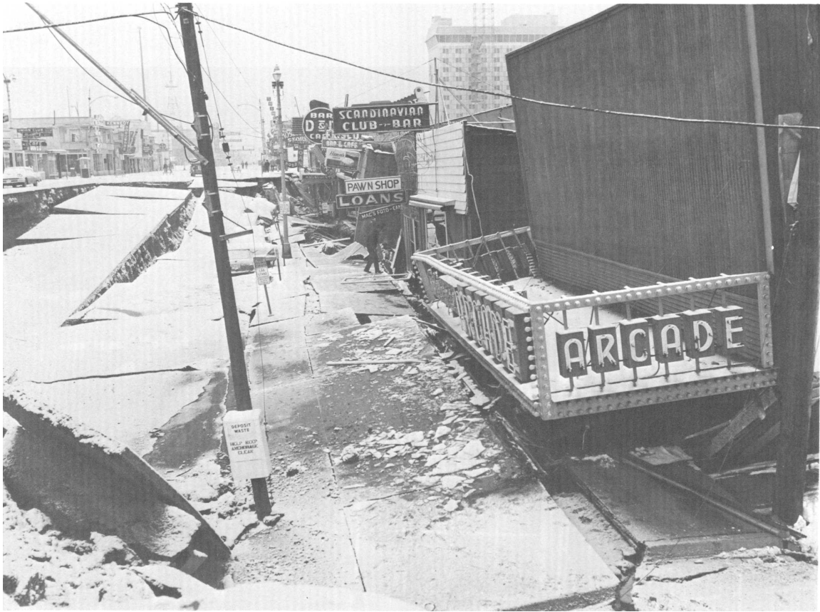
FIG. 4-1: Photograph at the head of the 4 th Avenue slide in Anchorage, Alaska, 1964 (Hansen 1971).
