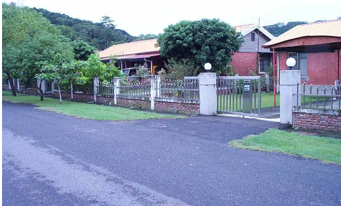
(f) 1-story buildings without evident ground failure or building settlement near the location of boring WAS-1
