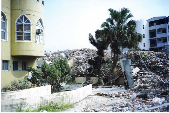
(d) 3-story building near the location of boring WAS-2 (photo by R. B. Seed)
