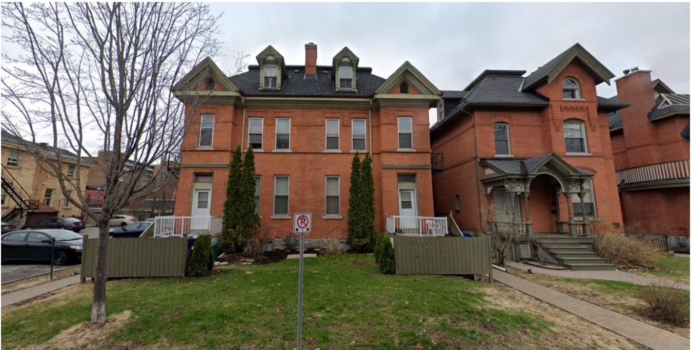
Figure 1: Subject Property frontage on Russell Avenue.
