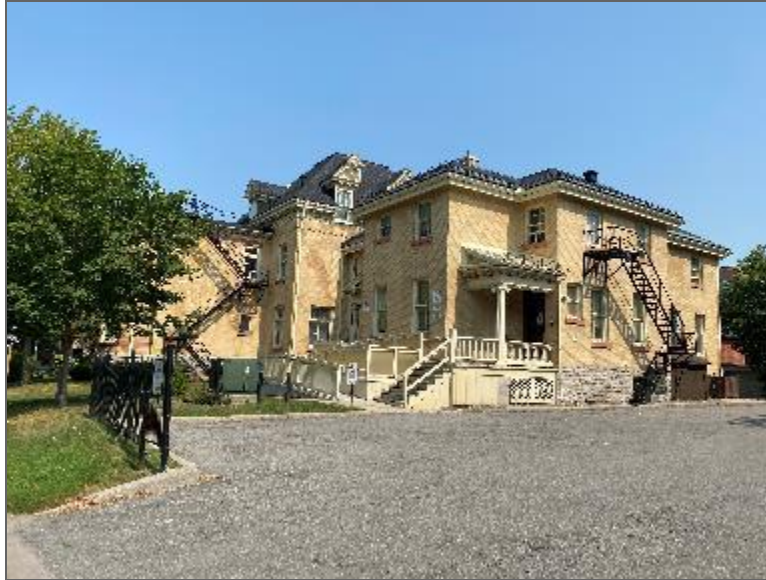
Photo 7 – Properties located northwest of the Phase One Property.
