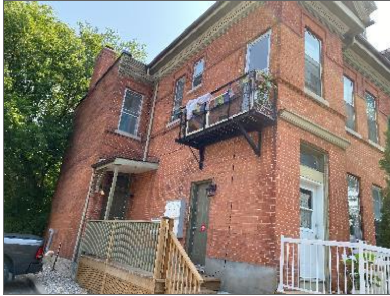
Photo 3 – Site Building (northwest elevation).
