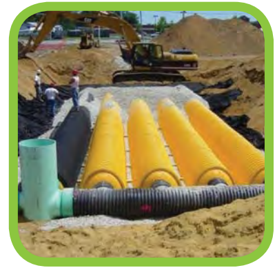
Looking down the Isolator Row PLUS from the manhole opening, ADS PLUS Fabric is shown between the chamber and stone base.
