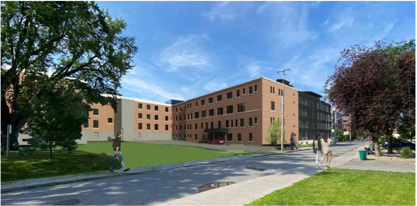
Figure 13. View along Springhurst Avenue from the northeast
