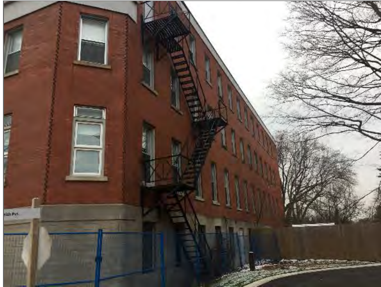
Photo 3 – Site Building (east elevation).
