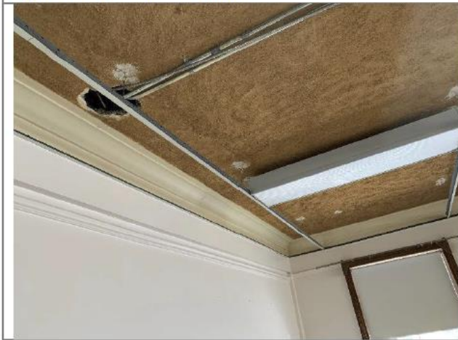
Figure 28: Room with ceiling system removed
