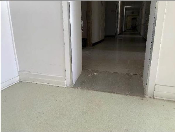
Figure 43: Ramp at floor elevation change
