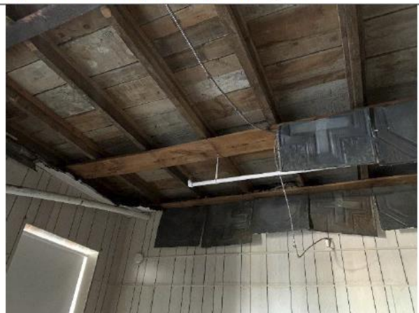
Figure 25: Exposed Ceiling revealing floor board, stripped ceiling finishes
