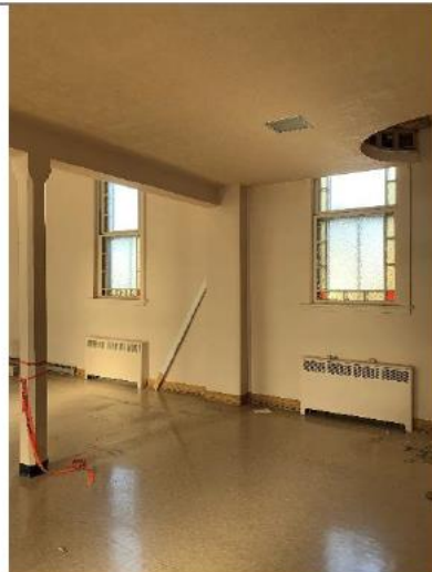
Figure 19: Removed circular stair at chapel
