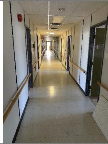
Figure 36: Care wing Hallway with parallel handrailing
