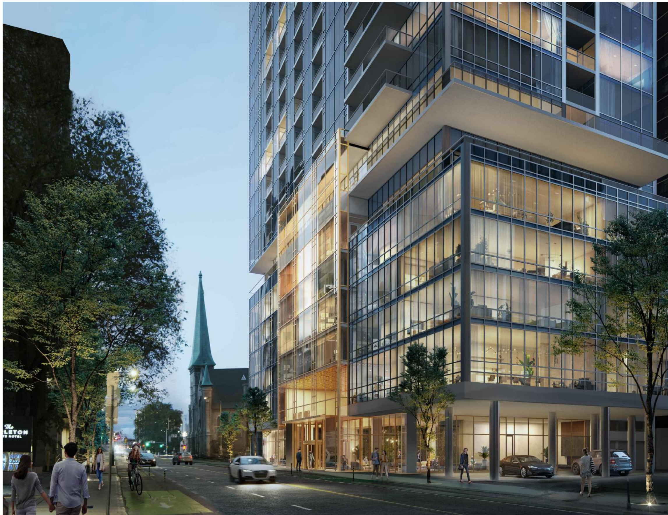
PEDESTRIAN VIEW LOOKING SOUTH EAST ACROSS STREET
