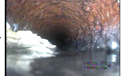
Figure#10: A view to the 50mm 12 o'clock connection at 11.8 meters from the top HALLWAY FLOOR CO.
