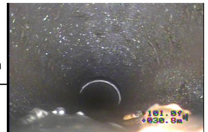
Figure#18: A view to the line deviation downwards at 30.0 meters from the top of HALLWAY FLOOR CO. Angular
