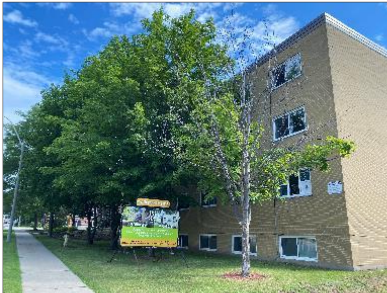
Photo 6 – Properties located north of the Site.
