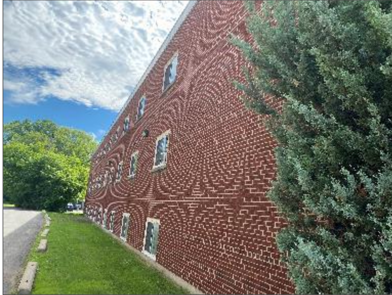
Photo 1 – Site Building (north elevation).
