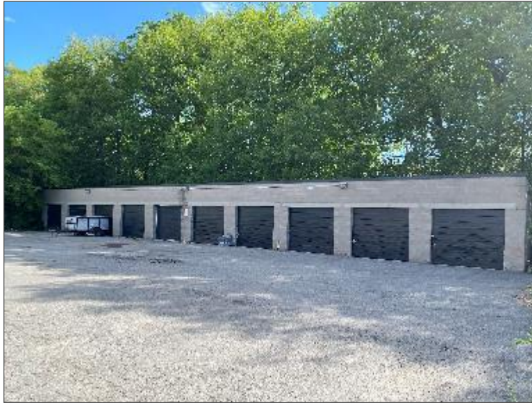
Photo 5 – Parking garage building on the east portion of the Site.
