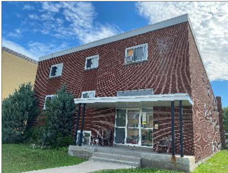
Photo 4 – Site Building (west elevation).
