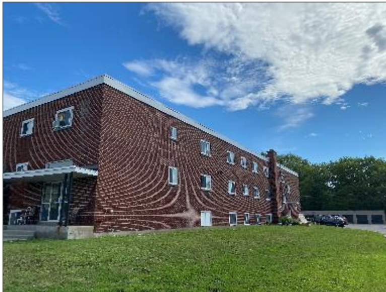
Photo 2 – Site Building (south elevation).
