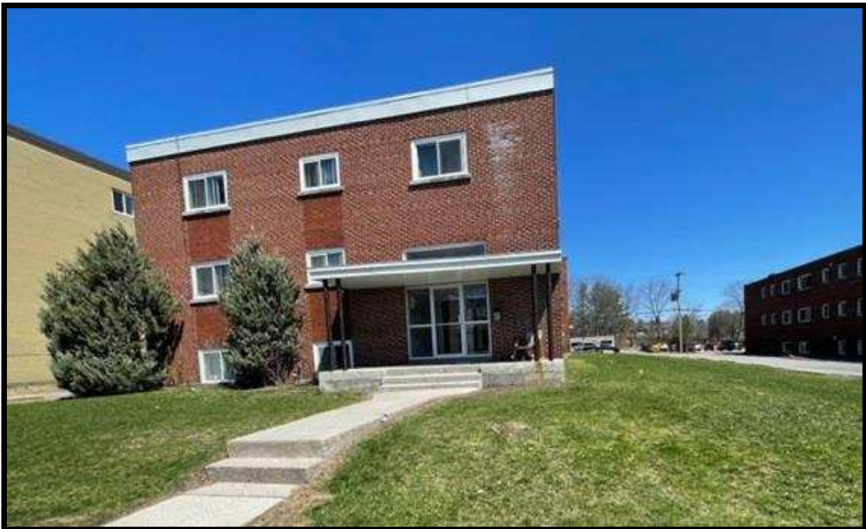
Photograph 2: View of the west side (or front face) of the subject building, looking east.
