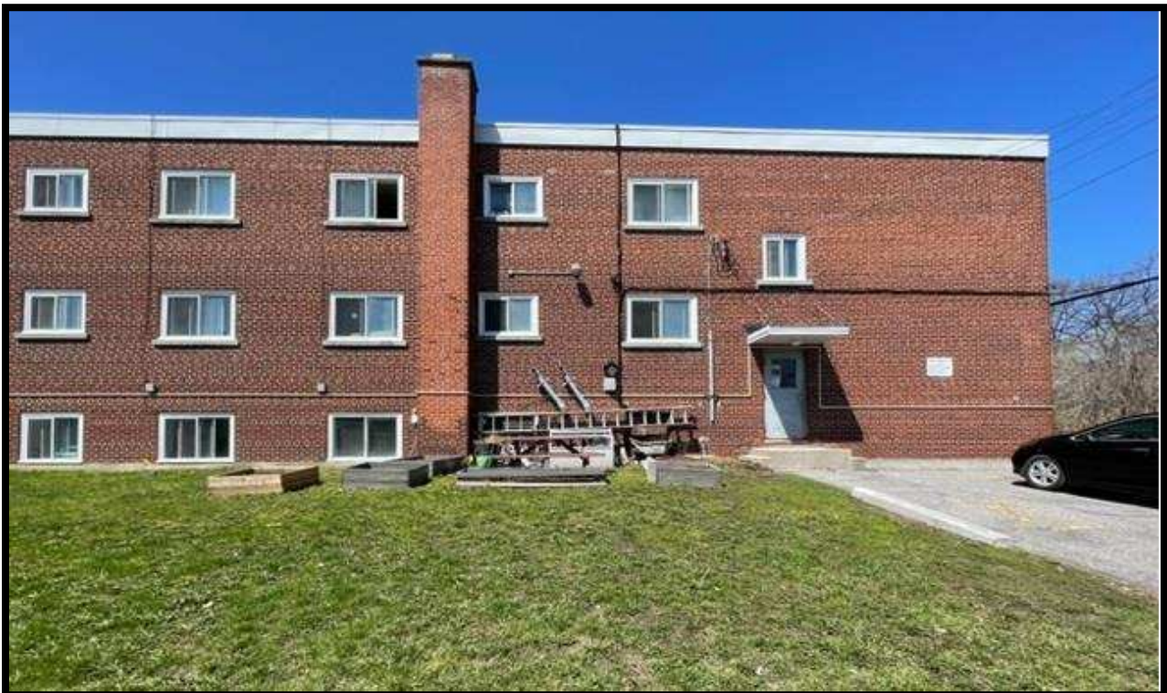
Photograph 4: South face of the subject building, looking north towards Montreal Road.
