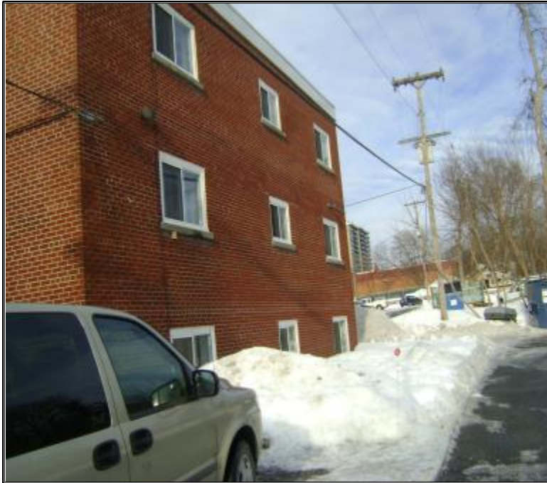
Photo 3 – General exterior view of the Site Building (east elevation).
