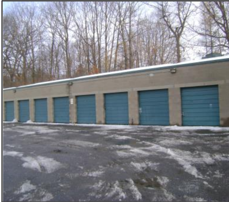
Photo 5 – General view of the parking garage located on the east portion of the Site.
