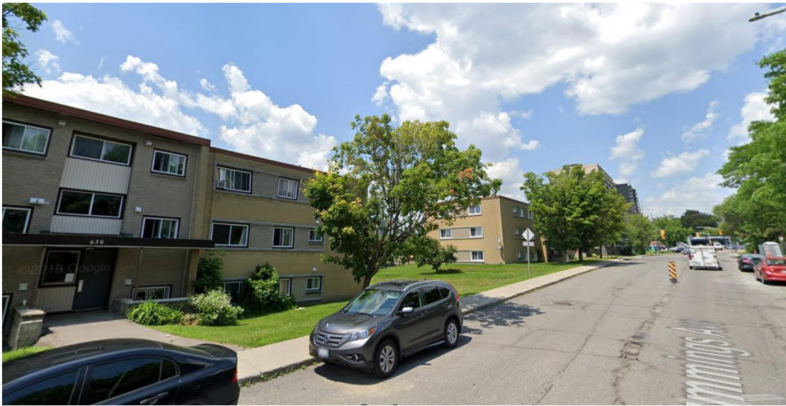
Photograph 5: Looking north along west side of Cummings Avenue towards Montreal Road.
