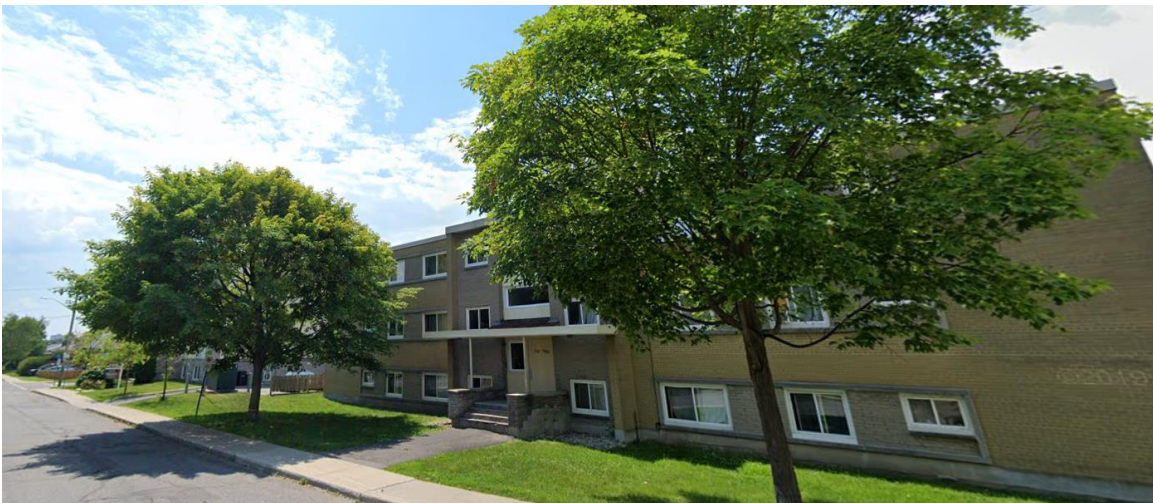
Photograph 3: Looking south along west side with 640 Cummings Avenue in the foreground.
