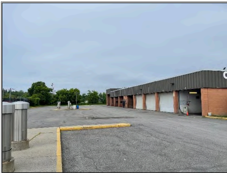
Photo 2 – Site Building (south elevation).
