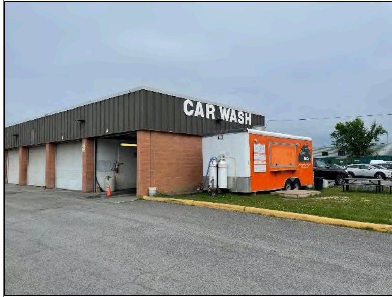
Photo 3 – Site Building and chip truck (east elevation).
