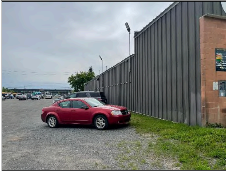
Photo 1 – Site Building (north elevation).
