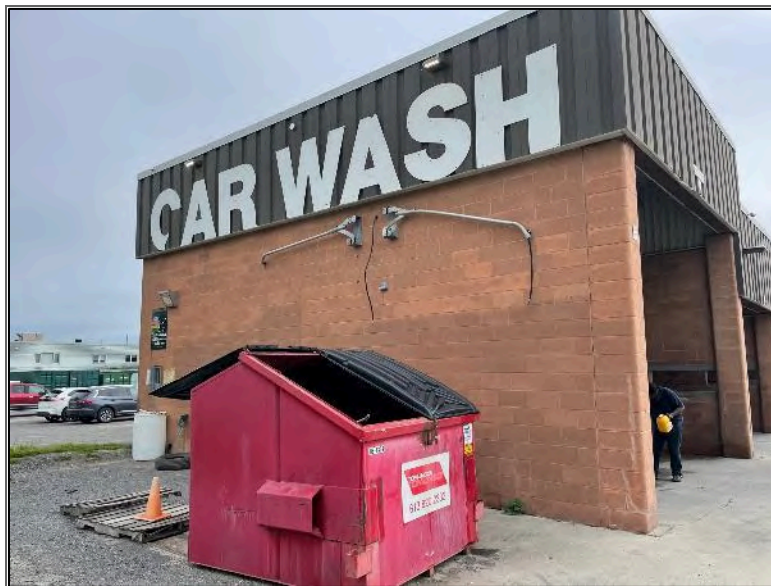
Photo 4 – Site Building (west elevation).
