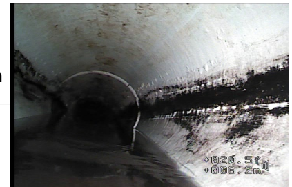
Figure#6: A view to the mm% of the pipe's surface area lost due to the deformed pipe at 6.6 meters from the
