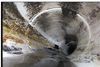
Figure#5: A view to the right line deviation at 5.2 meters from the top of STACKCO (RD1).
