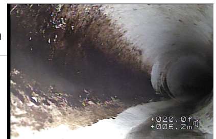
Figure#6: A view to the right line deviation at 6.2 meters from the top of STACKCO (RD1).
