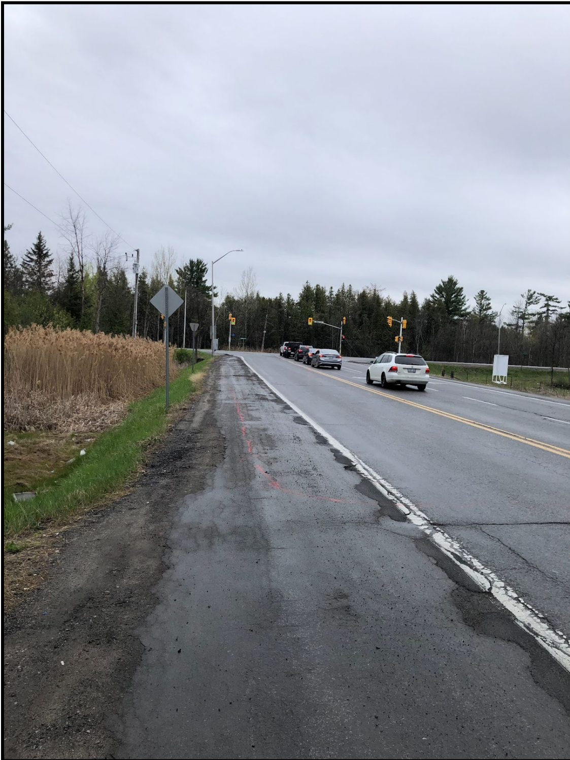
Site photo of Dunrobin Rd. looking south towards Dunrobin Rd. at March Rd.
