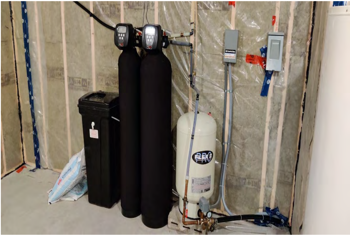
Photograph I8: Inside view of the basement
