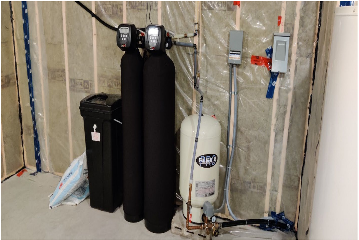
Photograph 18: Inside view of the basement
