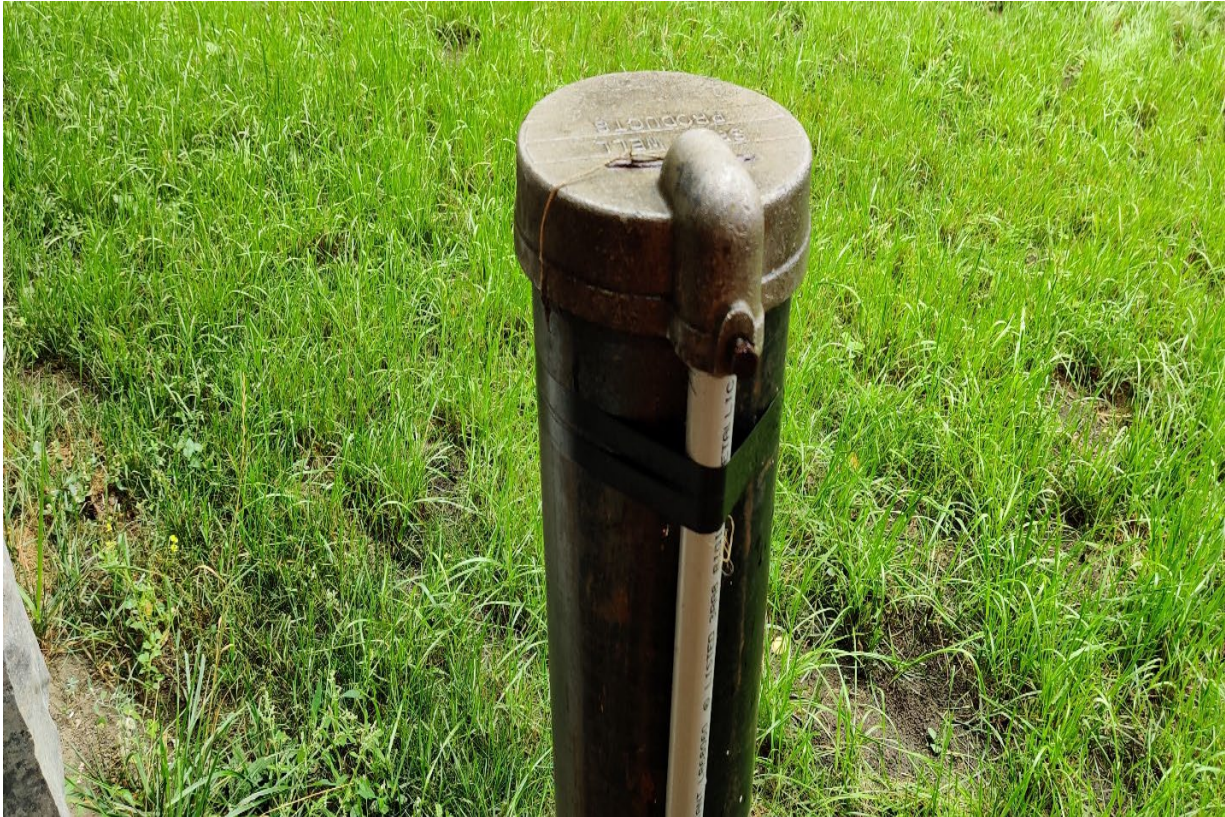
Photograph Plate I9: Water well on the subject property
