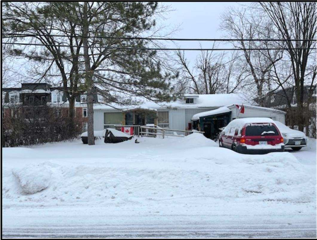
Photograph 1: The subject building at 2458 Cleroux, looking south.
