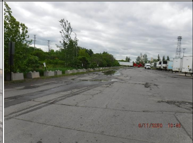
Photo 6: Existing Parking Lot
