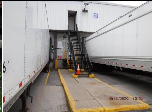
Photo 4: Existing Building Entrance
