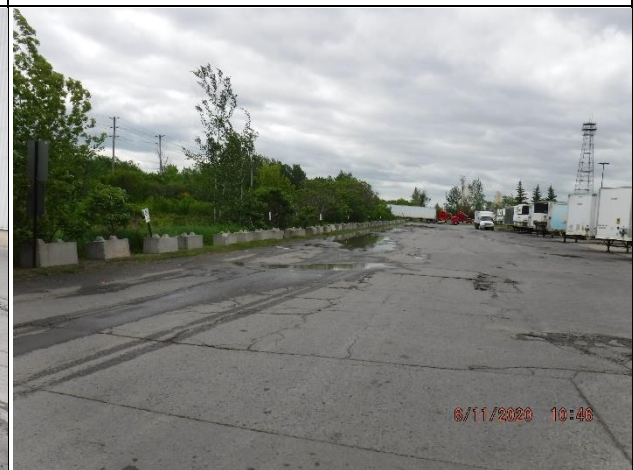
Photo 6: Existing Parking Lot
