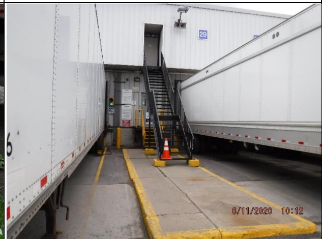
Photo 4: Existing Building Entrance
