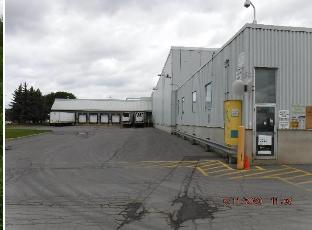
Photo 8: Existing Parking Lot
