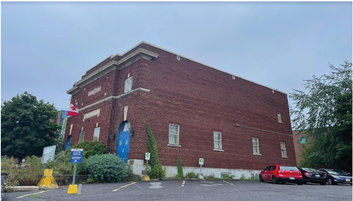
Figure 4: Westboro Masonic Hall, located immediately south of the subject site at the intersection of Churchill Avenue North and Byron Avenue
