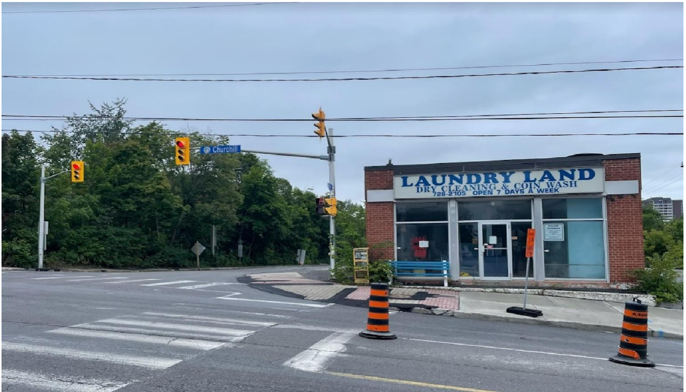
Figure 5: Subject site, looking west at Churchill Avenue North and Byron Avenue intersection
