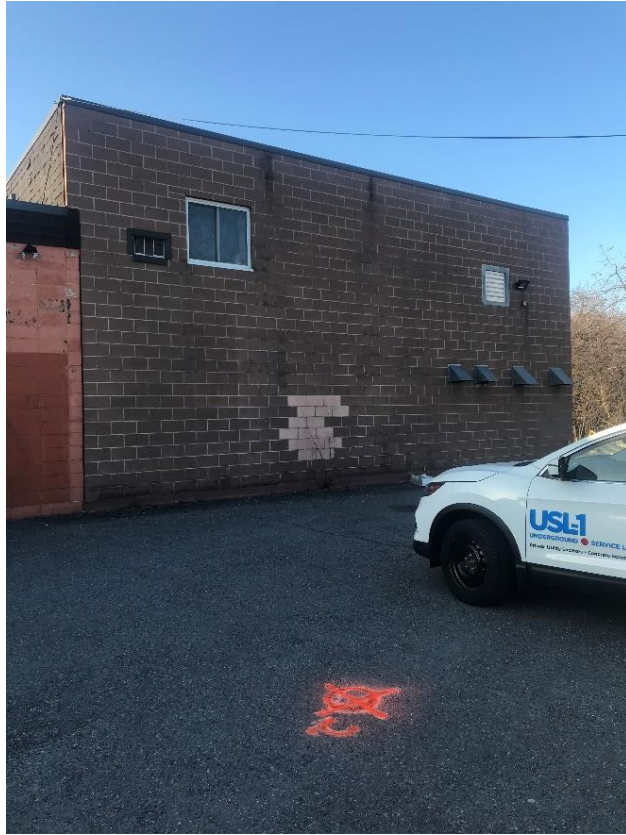
Photograph 5: Northwest face of Site building, facing east (April 6, 2021).
