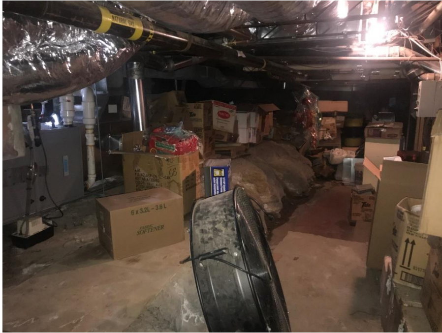
Photograph 23: Site building basement, storage (April 6, 2021).
