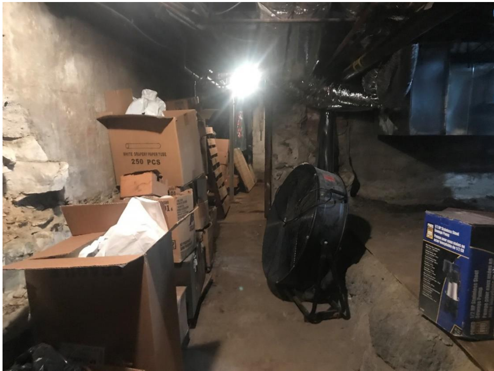
Photograph 22: Site building basement, storage (April 6, 2021).
