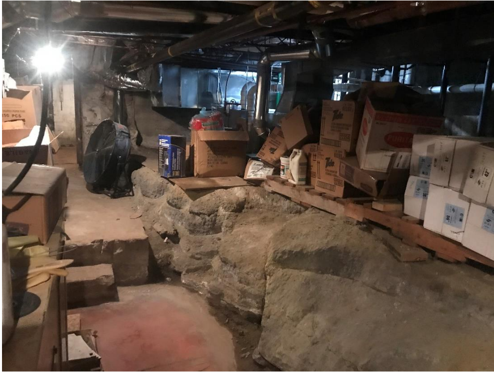
Photograph 21: Site building basement, storage (April 6, 2021).
