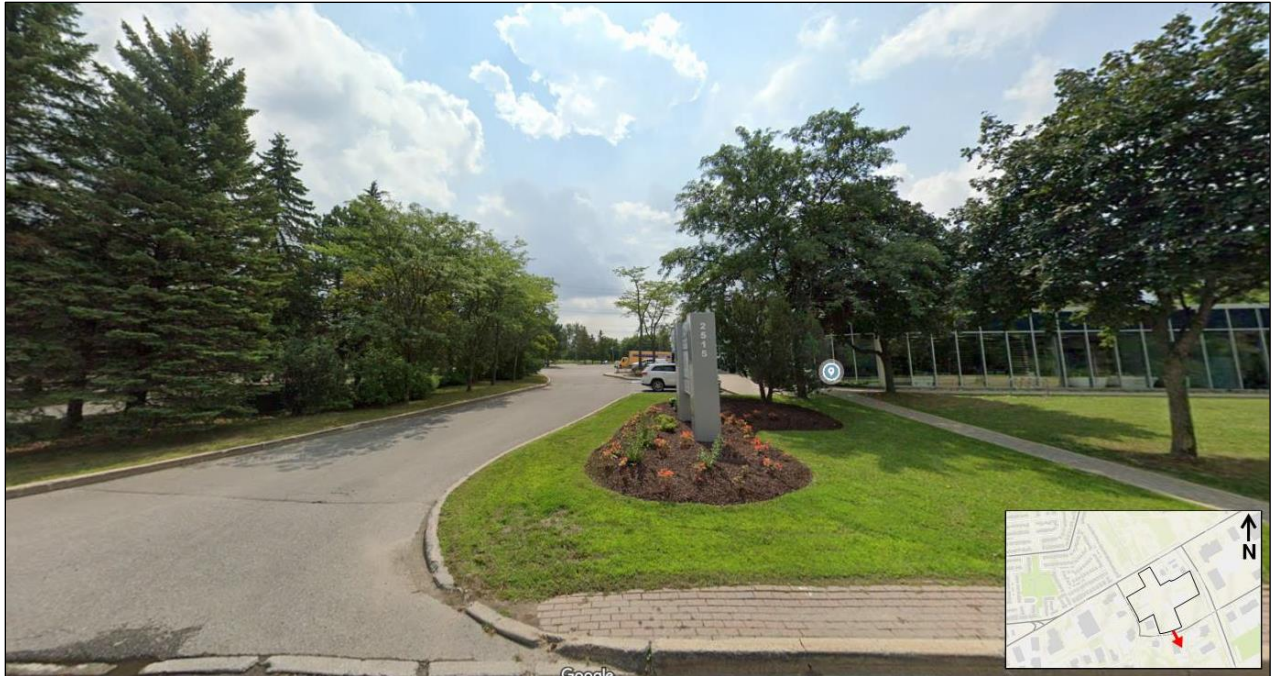
Figure 11: Looking south at the existing office building at 2515 St. Laurent Boulevard
