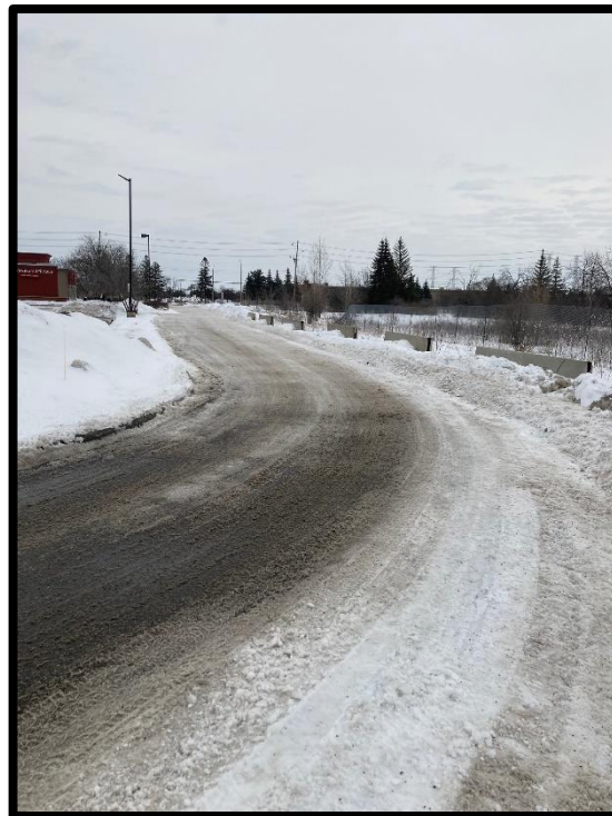
Photograph 4: View of the asphaltic concrete roadway on the 2990 Conroy Road portion of the Phase I Property, facing east.
