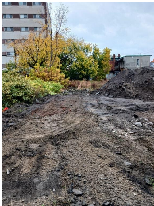
Image of surficial soil commencing excavation
