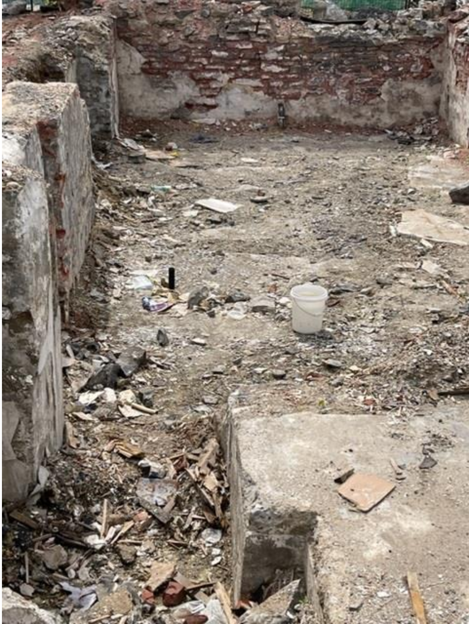
Image 3 - EXMW2 within the basement foundation
